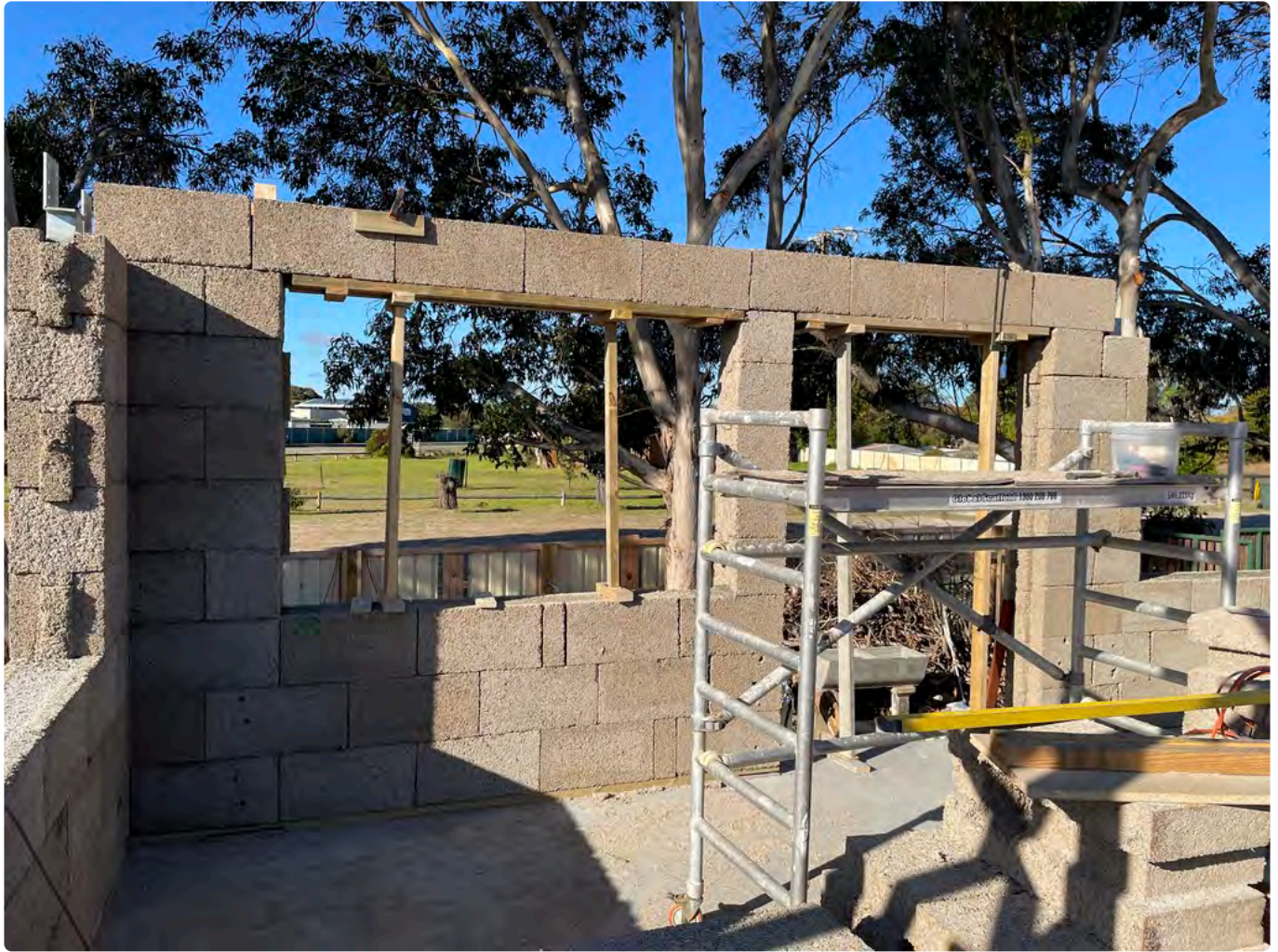
Timber lintel block supports.
